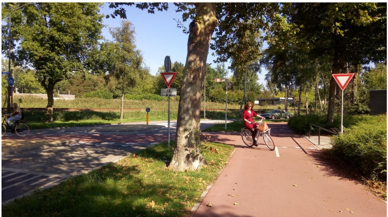
Figure 5. Because of insufficient curve radius at the connection of cycle tracks, the cyclist joining from the crossing will enter the part of the cycle track meant for traffic in the opposite direction.
