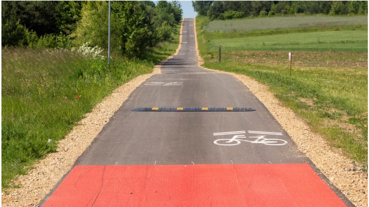
Figure 7. This obstacle, hidden behind a vertical curve for the cyclists coming from the opposite direction, was the cause of a serious accident. Photo credit: Agnieszka Fabiańczyk.
