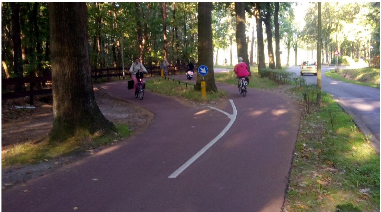
Figure 9. A bidirectional cycle track split into two unidirectional to ensure sufficient curve radius and sight distance without cutting the tree.
