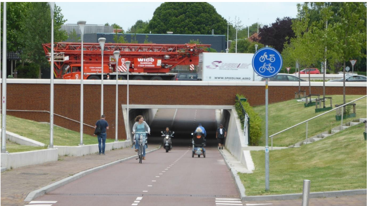
Figure 3. Cycle highways in the Dutch province of Gelderland are usually 4 m wide, cross major roads by tunnels and bridges, and cost between €300,000 and €1,800,000 per km.
