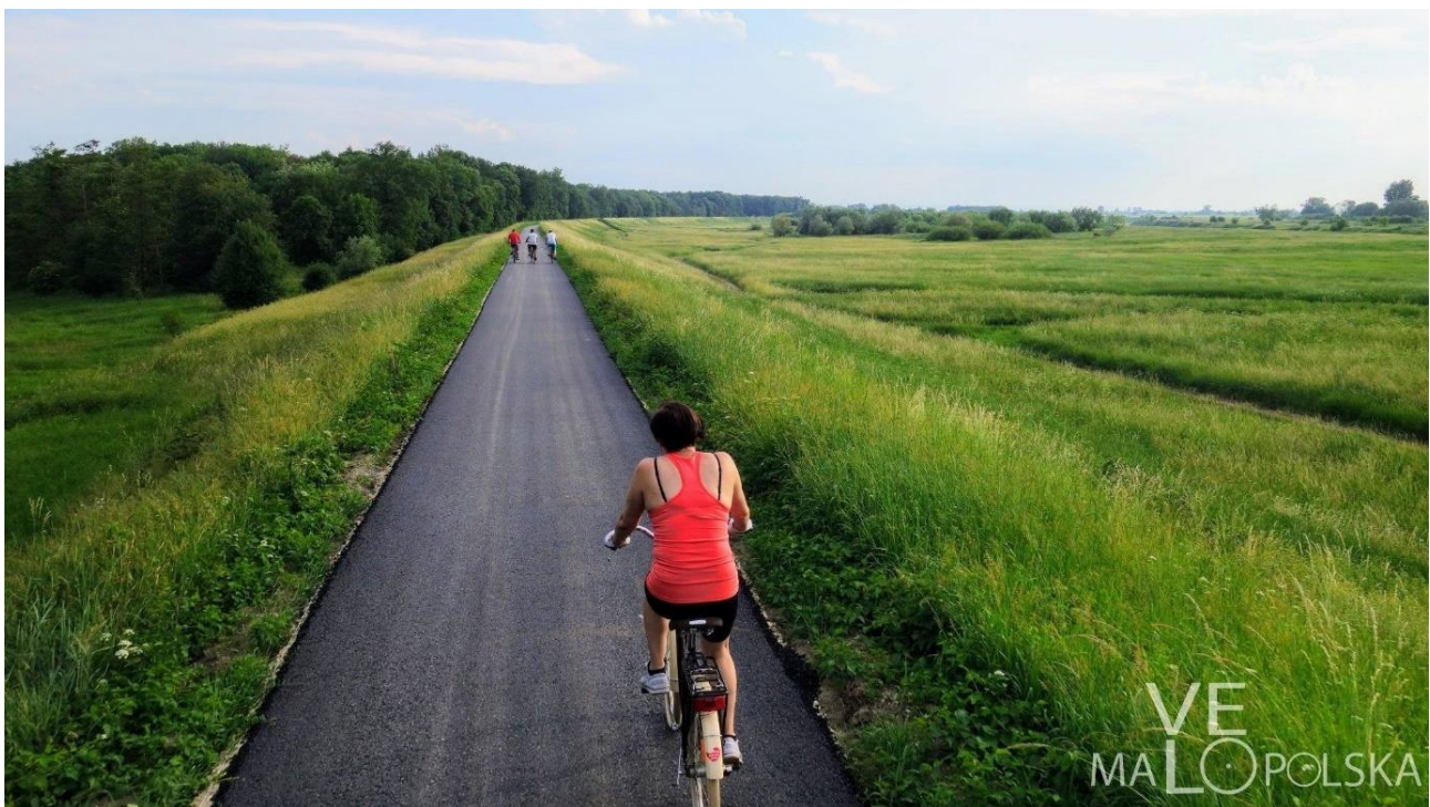
Figure 1. In greenfield conditions, a high-quality cycle track can be built for €50,000 per km. Photo credit: VeloMatopolska.
